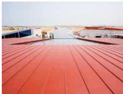
LEWIS® dry roof cassette with estimated weight 15 kg/m 2
