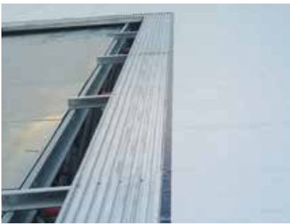
LEWIS® dry roof cassette with estimated weight 15 kg/m 2
